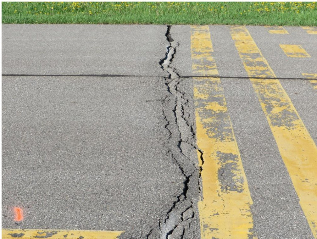
BDH PTA 001 (High-Severity L&T Crack – Sample Unit 151)
